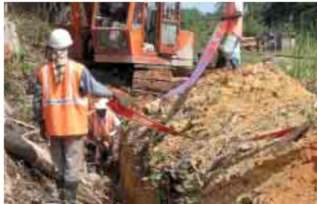
Fiber optic cable laying
