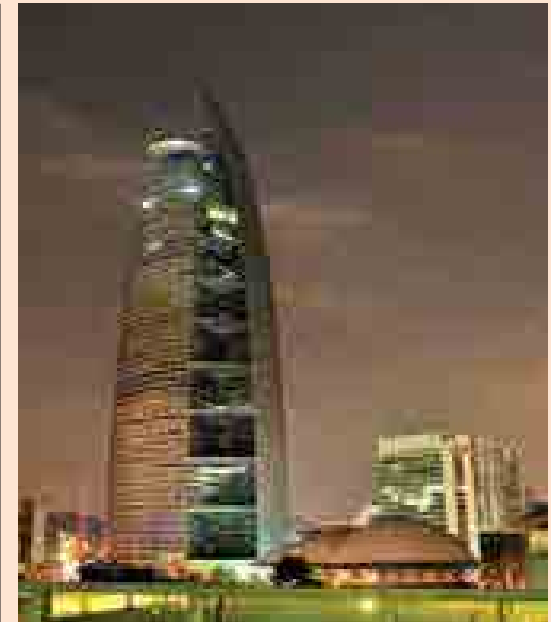
Menara TM is one of the most energy efficient buildings in the country.
