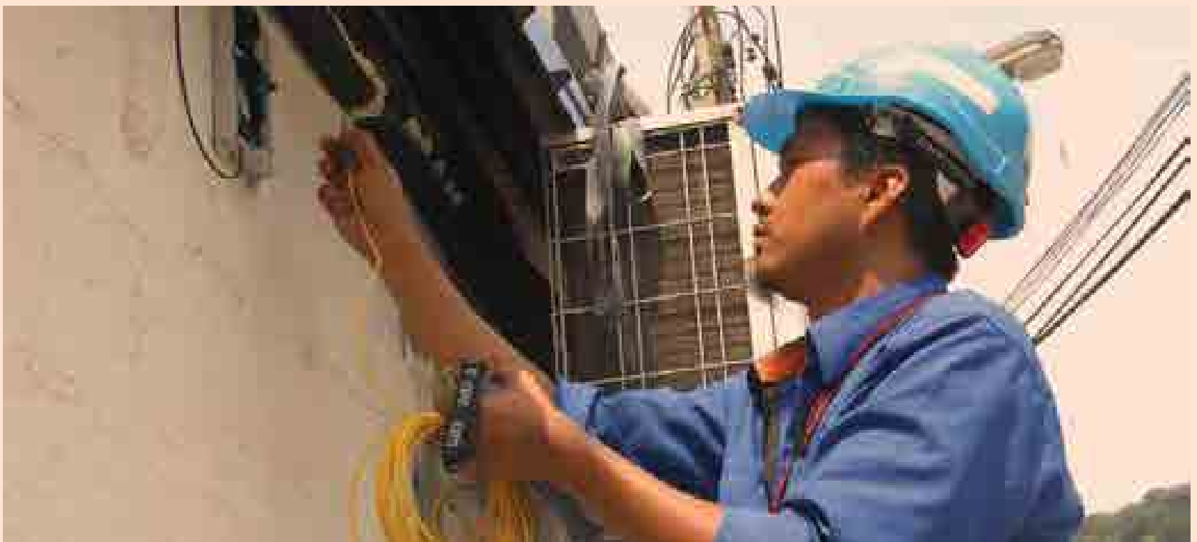
A technician completes Malaysia's first FTH installation, powered by TM's UniFi.
