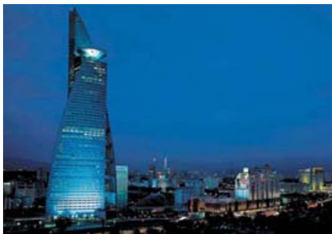
A Beacon on the KL Skyline – Menara TM
