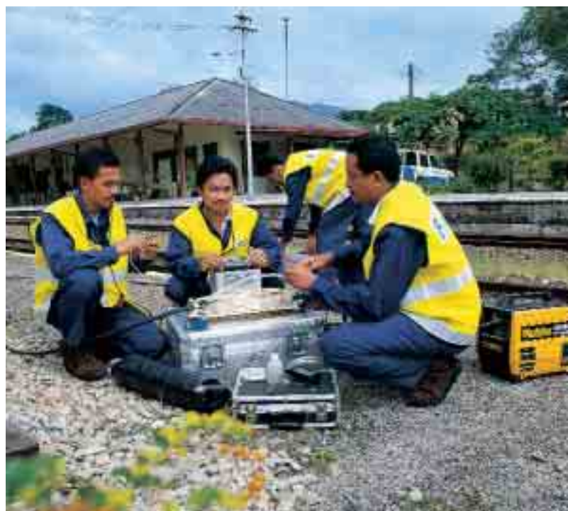
Fiberail – Malaysia's premier carrier-neutral wholesale network provider.
